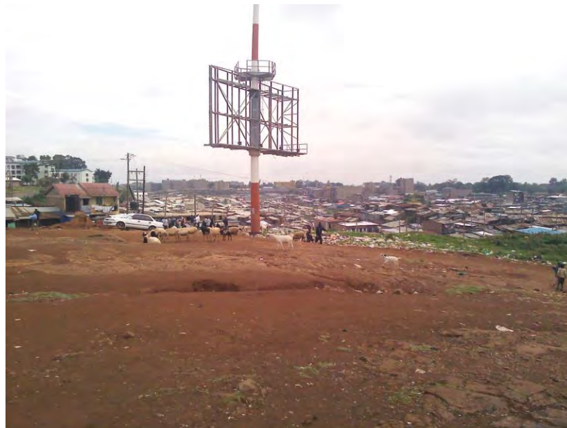
Figure 4. Open space with a light mast
