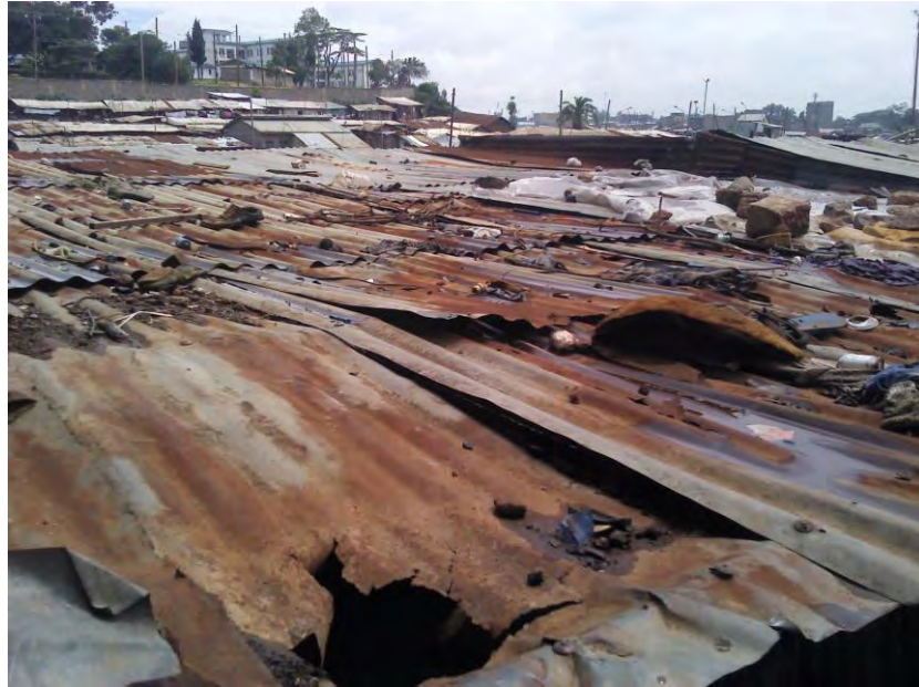
Fig.1. A shack structure from Mathare Valley seen from above
