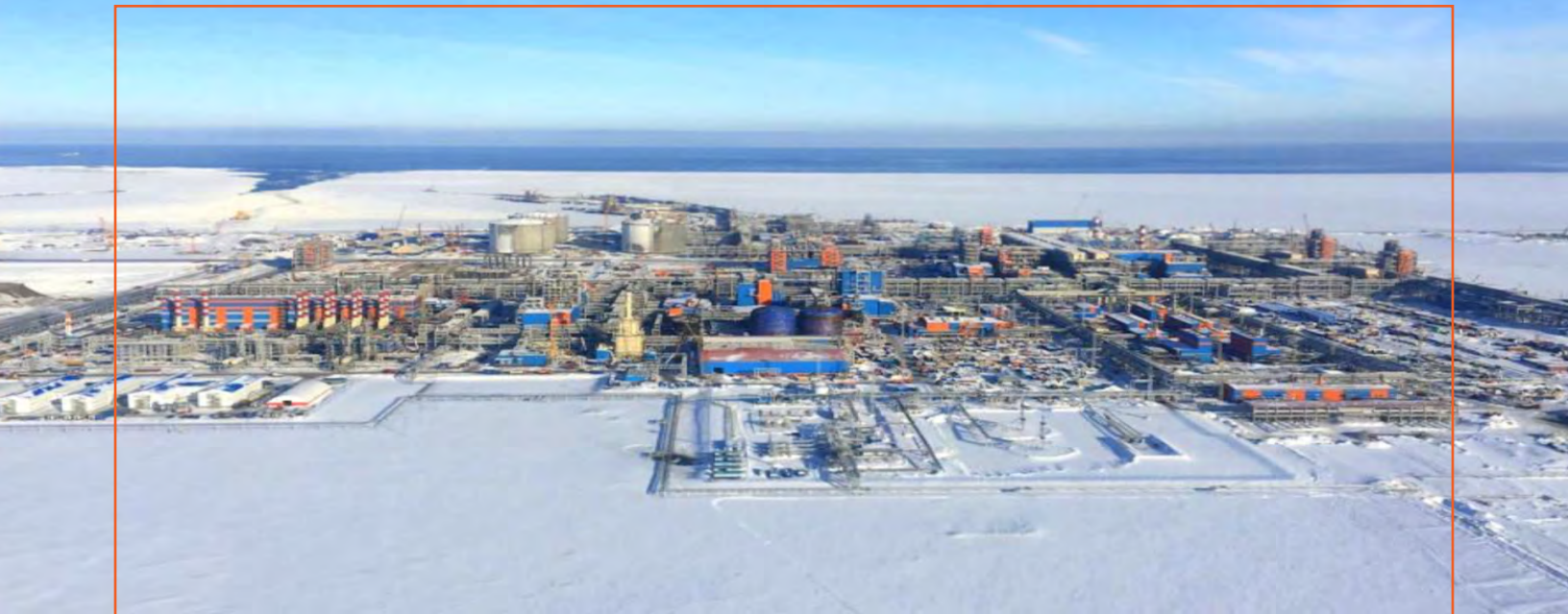
The Yamal Liquefied Natural Gas Plant, Sabetta, Russia. YAMAL LNG.
