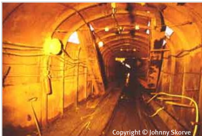
Fig. 13. Tunnel iron shelter
