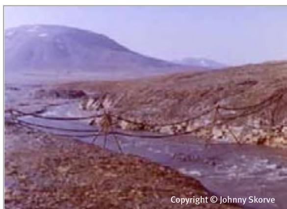
Fig. 5. Simple Zhuravlevka river crossing
